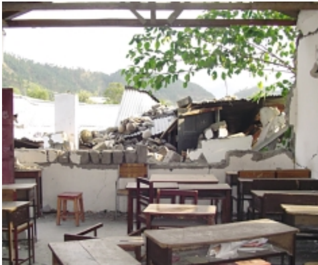
PAKISTAN: A school that was damaged by the South Asia earthquake.
